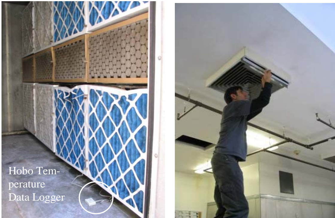
Figure 22. Temperature Loggers at the Filters in the MAU and at Kitchen's 4-way Diffuser
