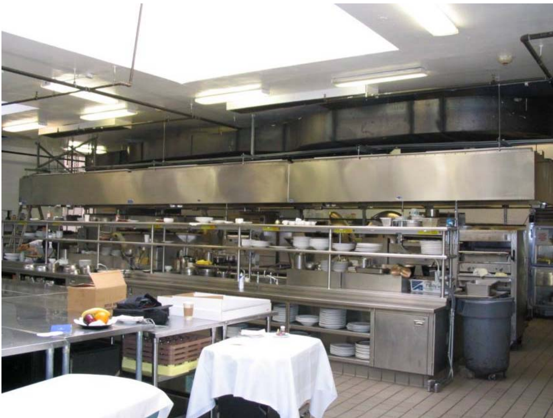
Figure 2. The Mark Hopkins Hotel Kitchen
