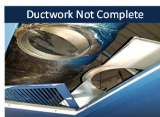
OA Dampers Not Installed
