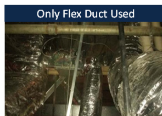
Ductwork Not Complete
