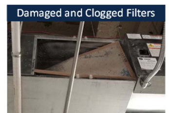
OA Dampers Not Installed
