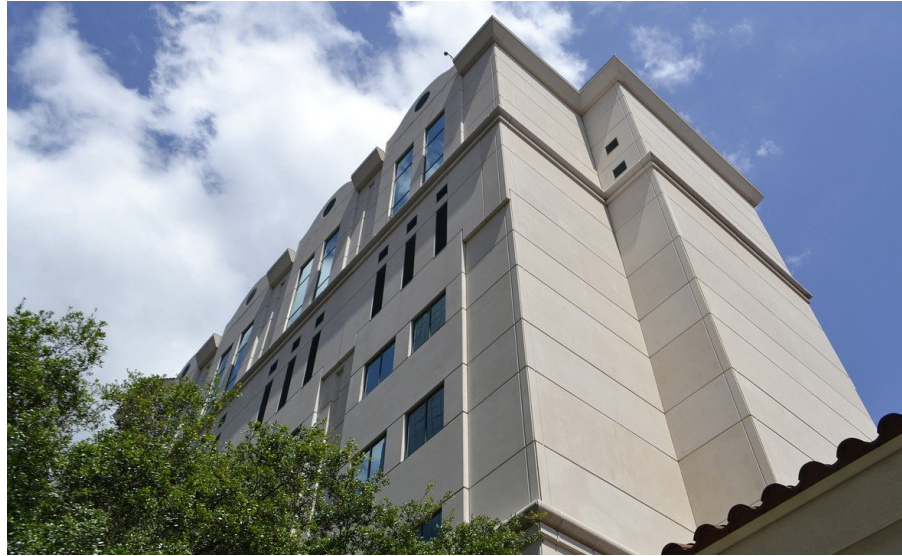
Melink's HVAC commissioning program verified plans for a medical office building. The second phase of the project includes rebalancing work.
