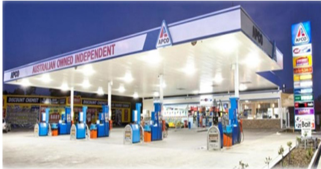
ecosense kitchen controls is installed in three petrol stations, reducing energy usage and operations costs.
