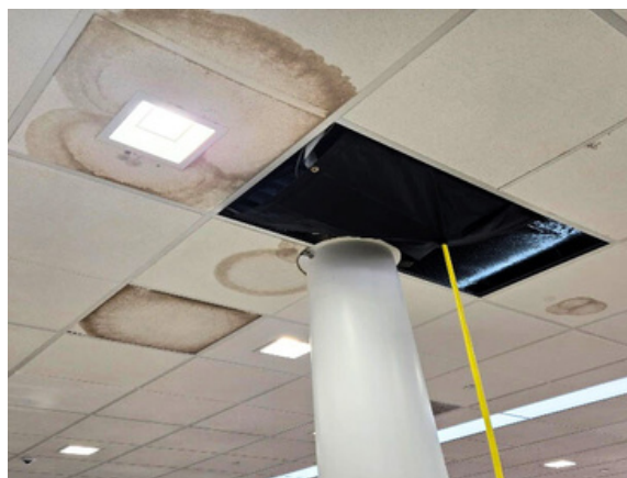
RTU condensation leak in store ceiling.
