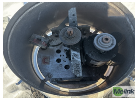
Exhaust fan with missing belt and not operational.
