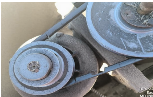
Exhaust fan belt has dry rot and is missing pieces.
