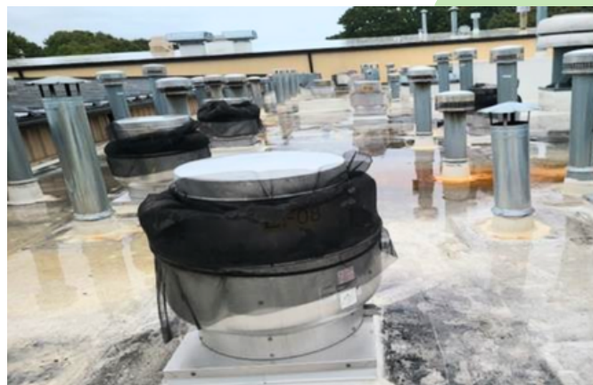
Exhaust fans have bonnets, trapping debris inside.
