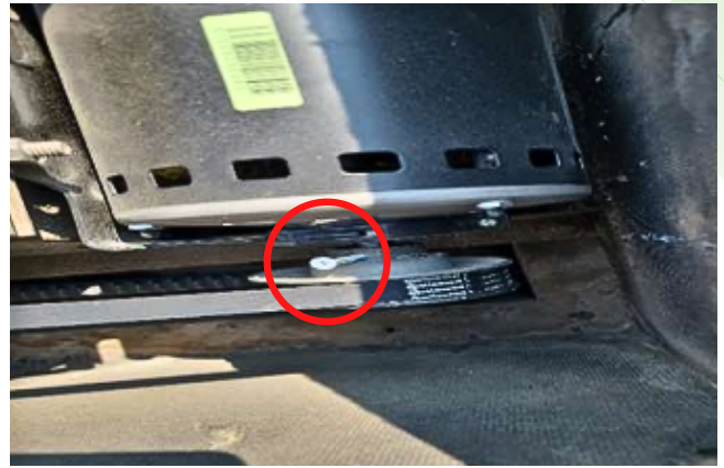
An exhaust fan motor pulley that is secured with a screw.
