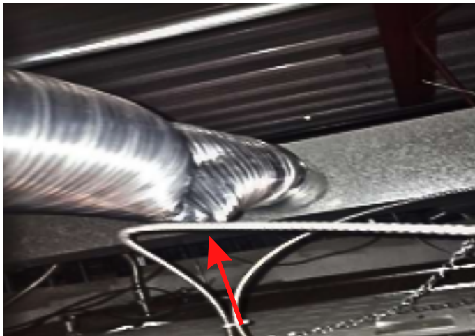
A section of rooftop unit ductwork that is dented and is not properly serving airflow to the connected diffuser.
