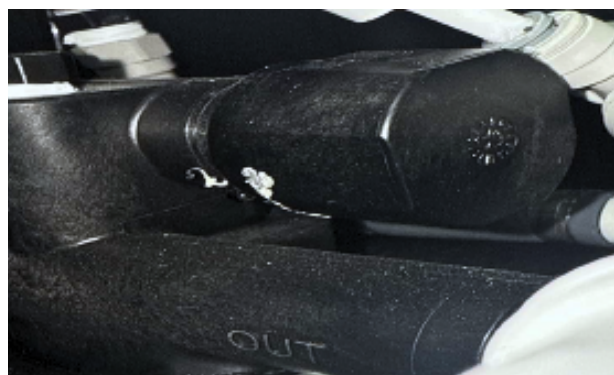
RO system is leaking.
