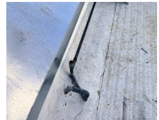
Condensate drain not connected.
