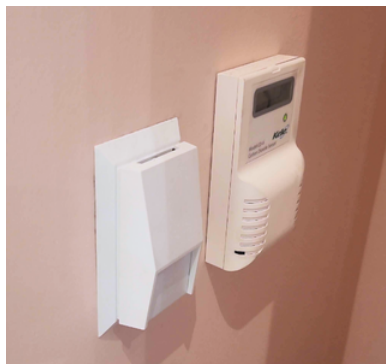
Remote sensor properly installed for RTU-3.
