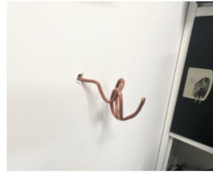
Missing temperature sensor for VAV.
