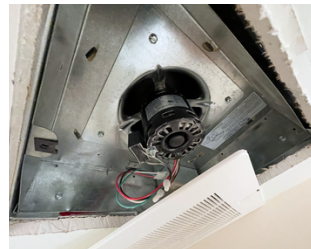
No speed controller installed on EF-1.
