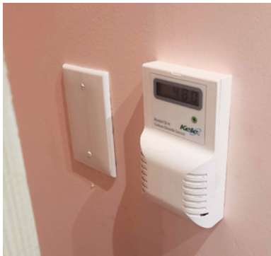
Remote sensor not installed for RTU-1.
